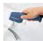
Cutting out small cable channels
